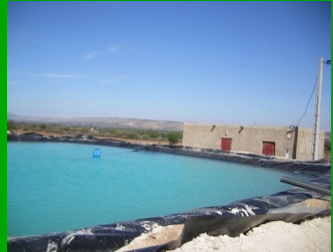
Installation of The PET membrane and filling of the bassin
